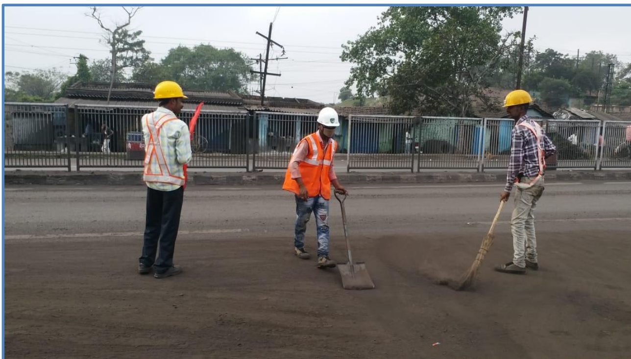
Picture 3 – Manual Sweeping of Public Road
