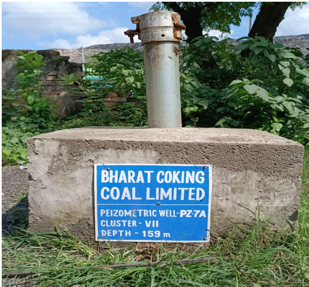
Picture 12 – Piezometer well
