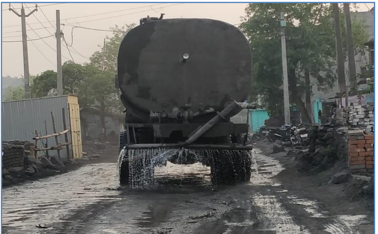
Picture 2 – Water Sprinkling on Transportation Road
